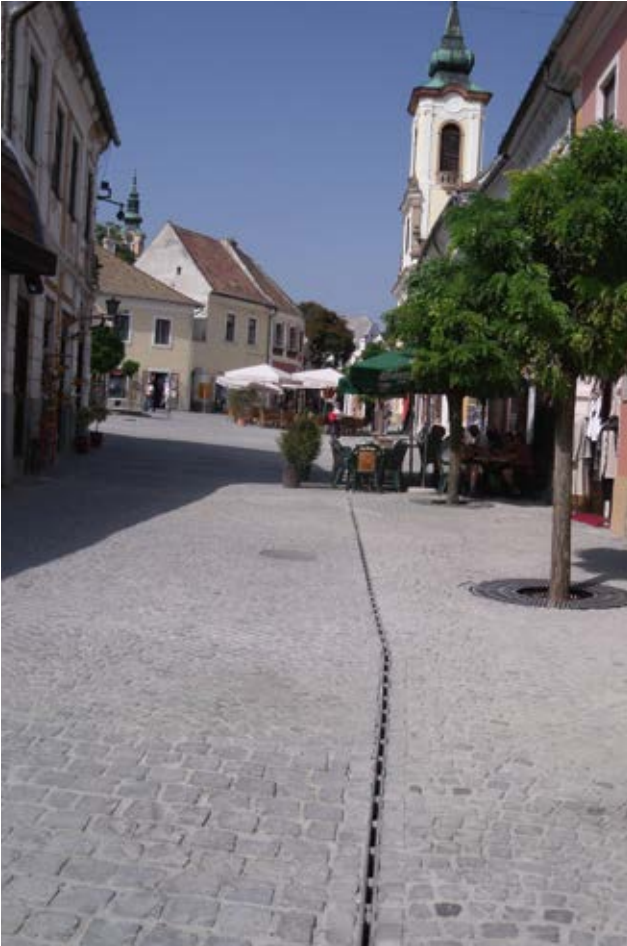
Renovation city center Szentendre, Hungary
