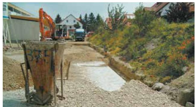
Laying the covering layers in the front-dumping method to allow vehicles to drive on the structure.
