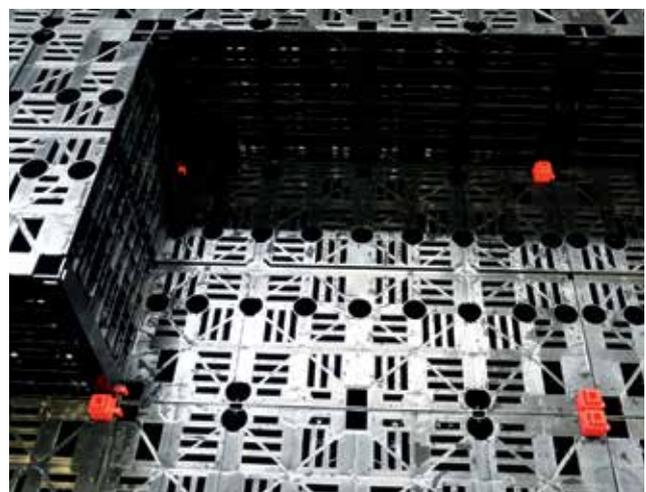
Shearing protection by means of adapter, 1 piece per DRAINFIX BLOC Size 1 in the surface
