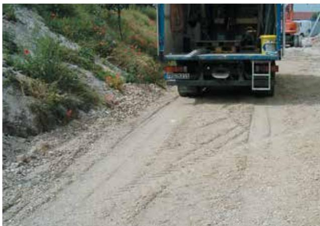
When the covering layer has reached a thickness of 50 cm it can support HGV of 12 t gross vehicle weight rating.
