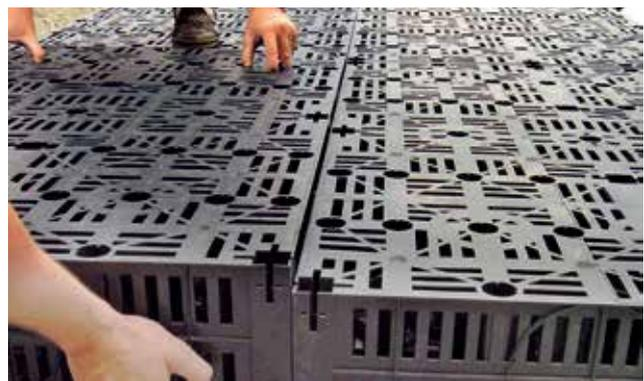
D Lower the DRAINFIX BLOC again and both sides of the block will be securely linked with resistance against thrust.
