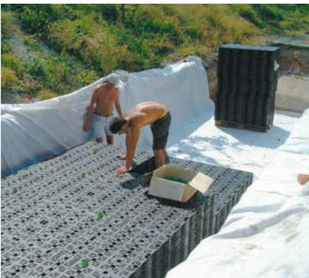
Laying several layers with connection adapter
